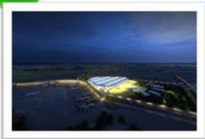
Mumbai Int'l Airport – Fixed Link Bridge RM26m
