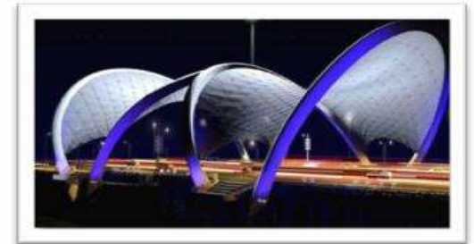
Lusail Expressway – NCC Gateway Arch RM14m
