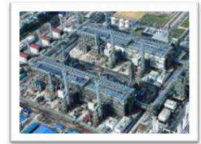
LNG Train 9 Project, Pipe Rack Structure RM19m
